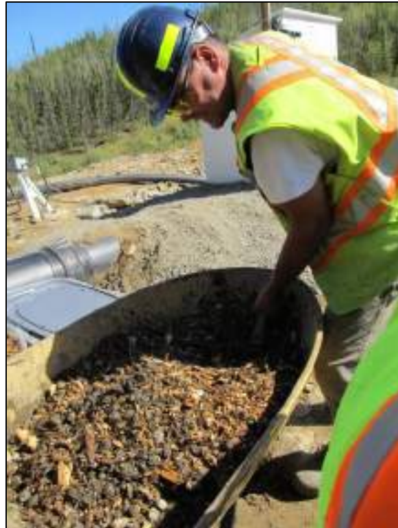
Figure 4. Bioreactors substrate mixture preparation.
